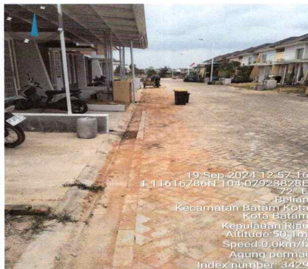
PAVING BLOK FINISING
