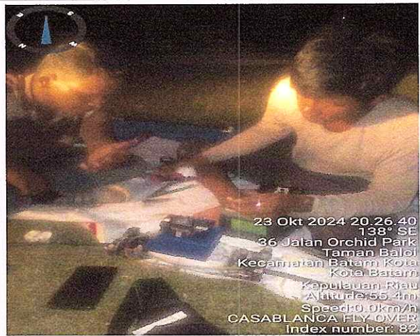
SPLICING KABEL RUSAK
